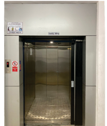
Traction Counter weight Goods Lift Cap : 500 Kg to 5 Ton
