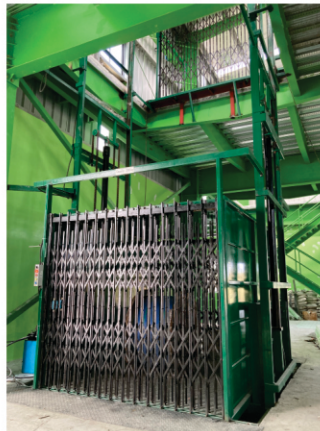
Double Mast Hydraulic Goods Lift Cap: 500 Kg to 5 Ton
